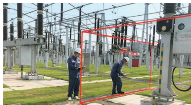
FIG 02 Working Site of Substation Personnel
